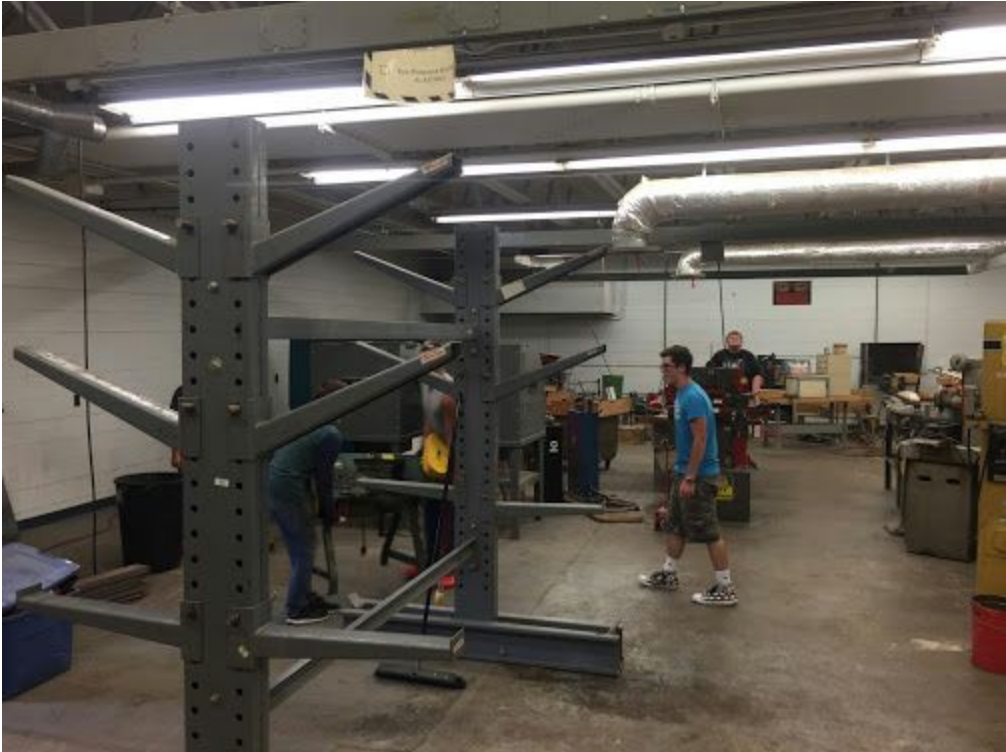
“During” or photos of the renovation process:
